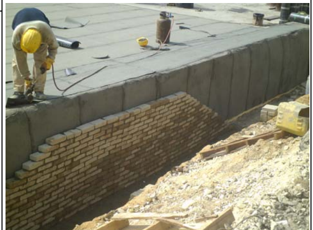
Construction site - Cairo Metro Line 3
