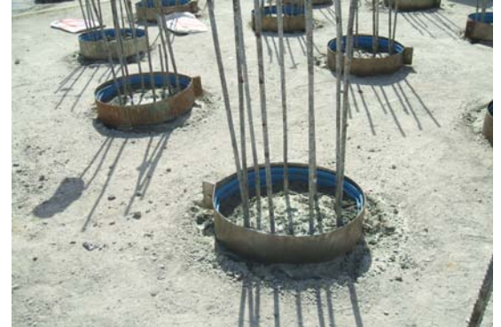
Construction site City Light Project
