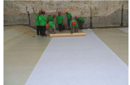
Construction site - Cairo Metro Line 3
